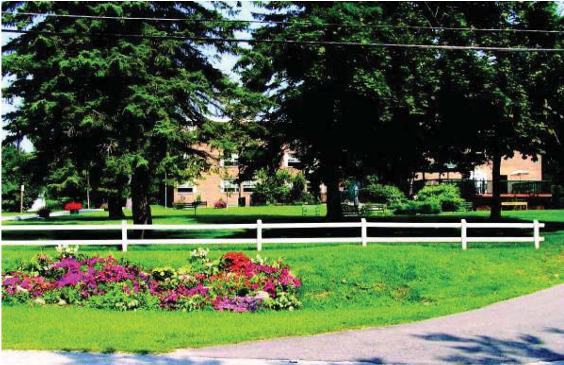
Figure I- 12: Rosebank Villa (Side View)
