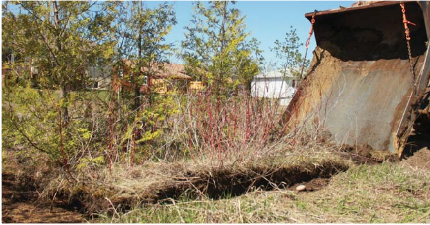
The slab technique of transplanting has been used in several other projects.
